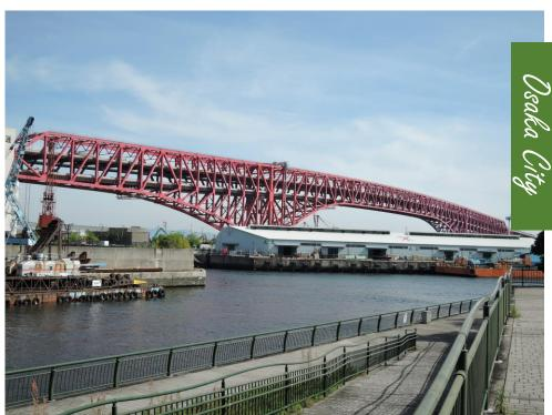
Minato Ohashi Bridge was completed in 1974 and has a total length of 980m. It is Japan's longest truss bridge and is one of the most distinctive landmarks in the Osaka Port area. You can see the full view of Minato Ohashi Bridge from the Hydrophilic seawall. There is a Chikko Akarengasoko (Red Brick Warehouse) near the Hydrophilic seawall. It has a history of about 100 years, so you can enjoy the atmosphere of the port town.
