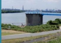
The intake tower takes water from the Yodogawa and supplies it to the water treatment plant. The facility helps us realize that we live with the water from the Yodogawa.
